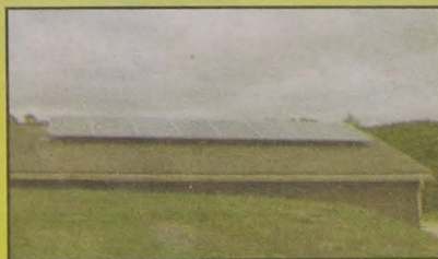
Seed Savers Exchange, Decorah 8 Sharp 230 watt panels and 8 Enphase inverters
