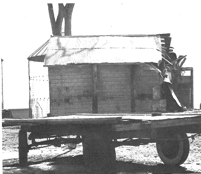
LEFT An old hayrack and a semi-demolished shed were parts of the farm before renovation began.
