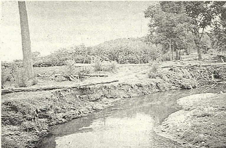
The project site before shaping and placement of rip-rap.
