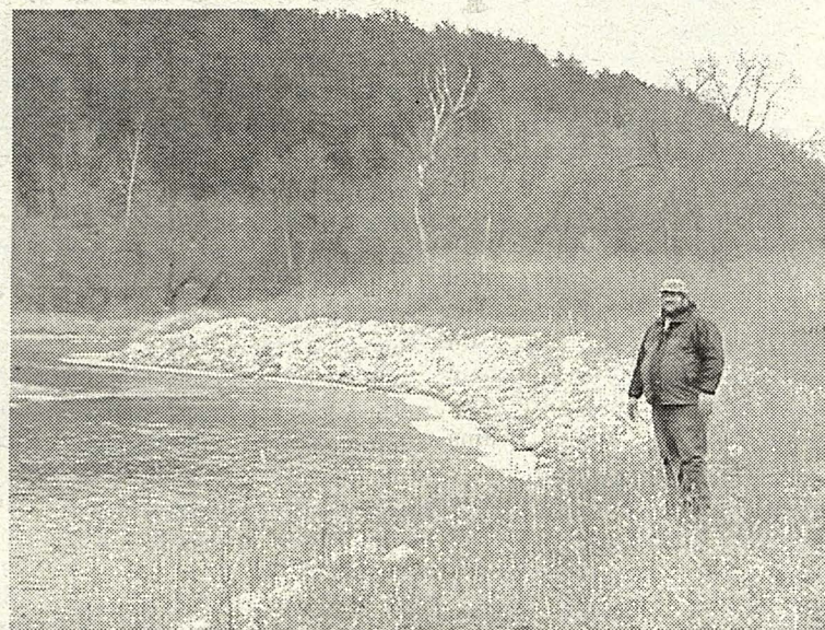
In the spring of 2001 after the construction was completed the water began to rise as usual but not to record levels. Neil said, "Not a stone was moved and the riprap prevent any further erosion."
