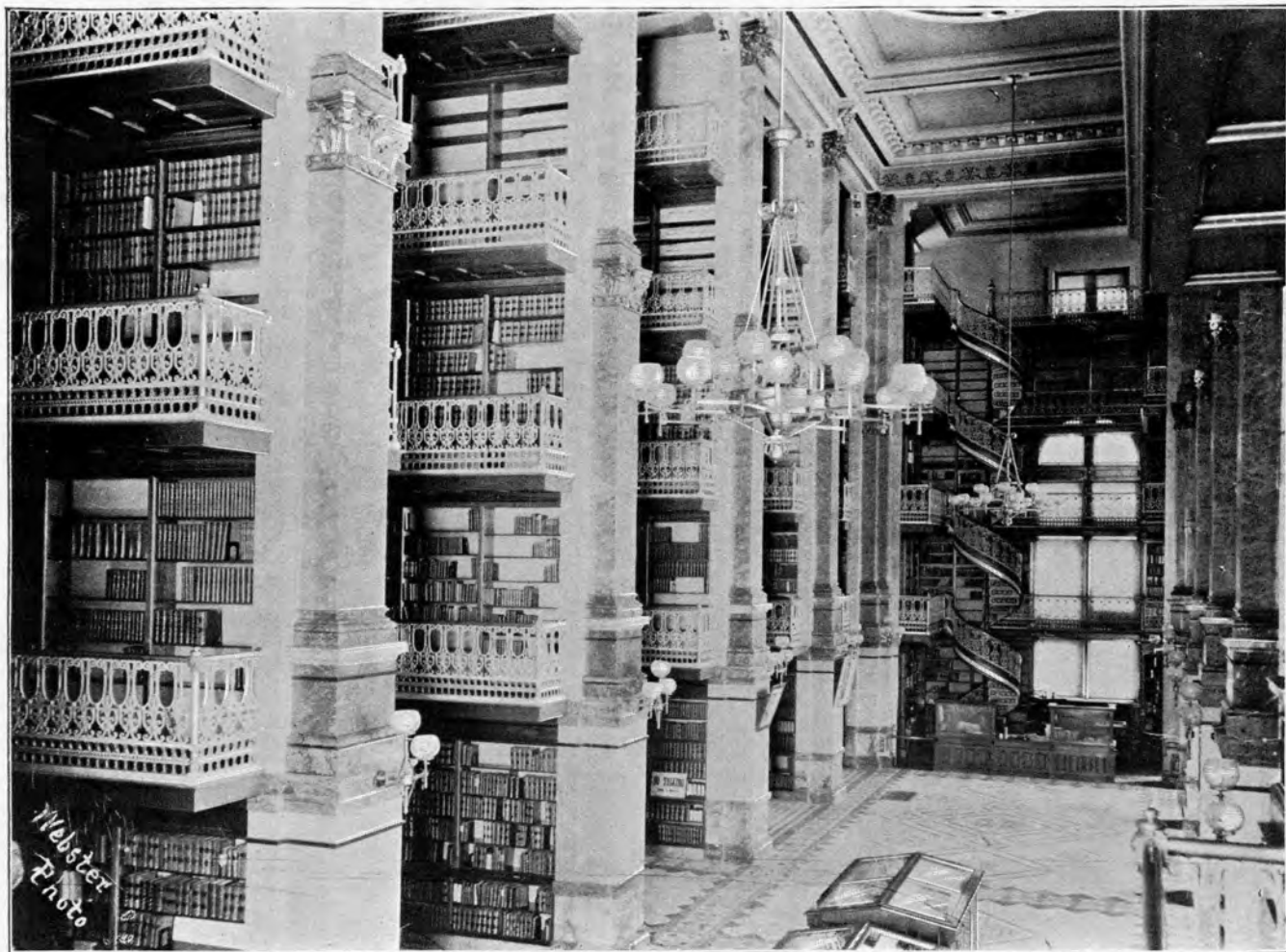
INTERIOR VIEW OF STATE LIBRARY—FROM NORTH GALLERY.
