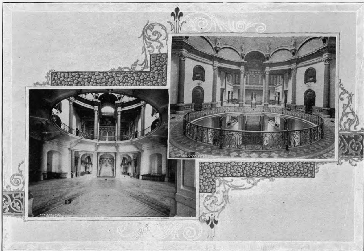
View from First Floor.
