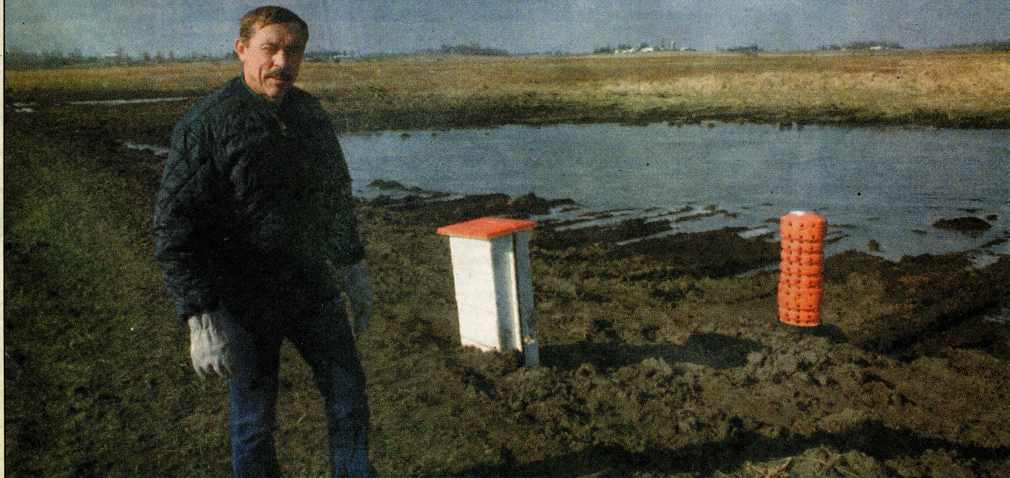
Waterloo firefighter Bob Boeck, shown standing on a newly constructed 5-foot dike, has spent five years restoring a 30-acre wetland north of the city. When the snow melts next spring, the water contained by the dike will be three to four feet deep. The structures at right are connected to an underground spillway and enable Boeck to control the water level, so that the area does not flood.
