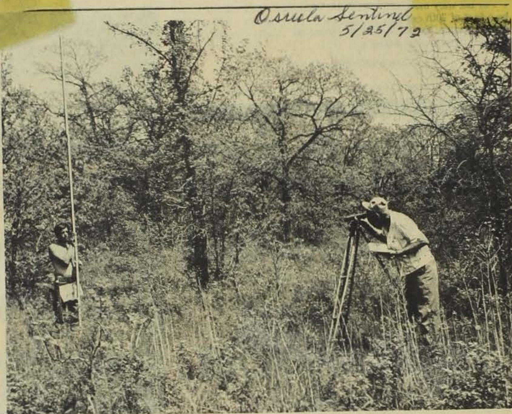
WHITE BREAST WATERSHED: Surveying in the White Breast Watershed has been progressing rapidly during the past three weeks. Jim Fluke, survey party leader, and Mark Cooper are shown as they move through a wooded area approximately three miles southeast of Osceola. Elevations are being established in the watershed area so that
