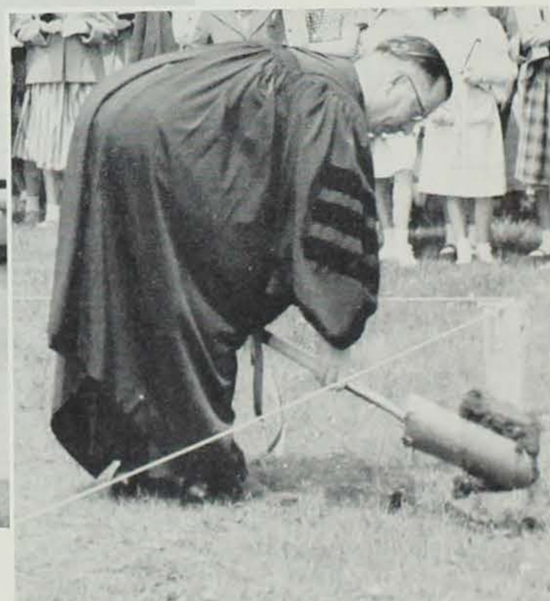
Ground Breaking May 17, 1953
