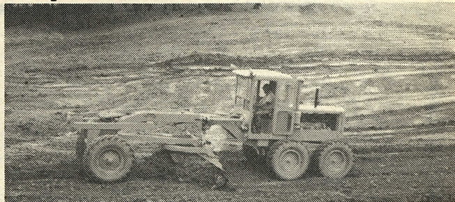
There was a lot of grading to do on a 3.5 acre pond Jim Bixler built in September. Dan Nietfeldt, Wheatland, was contracted for the grading. The project moved 7,200 cubic yards of soil.
