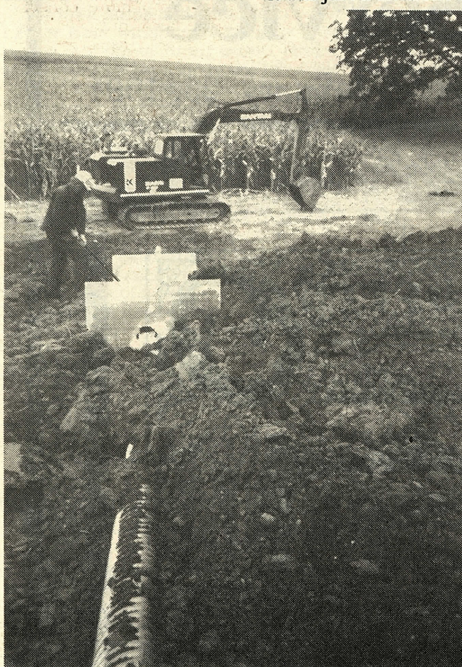
A large piece of equipment sits idle while 70 feet of overflow pipe is checked before being backfilled.
