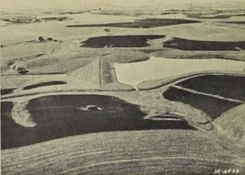
Detention Structure on the Walter Mortenson Farm in the completed Mortenson Watershed.
