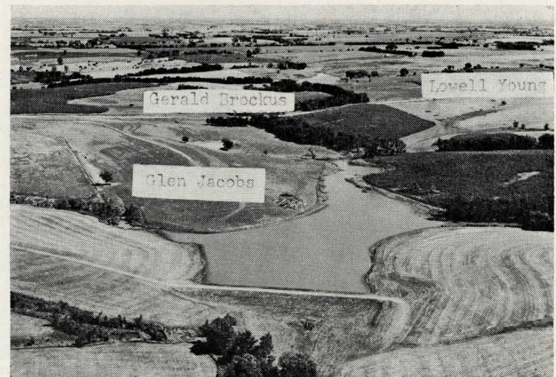
Grade stabilization structure B-8, Moulton Watershed, located on the Glen Jacobs farm 2\frac{1}{2} mi. northwest of Moulton. In the upper right, between the Jacobs and Lowell Young farms, a waterway (B-19) was also shaped and seeded with Public Law-566 funds.
