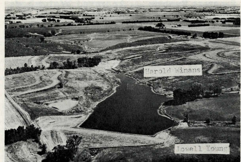
Grade stabilization structure B-2 in Moulton Watershed located on the Harold Winans and Lowell Young farms 2\frac{1}{2} mi. northwest of Moulton. Shown in the left foreground is a Pittman-Robertson wildlife planting which was installed by the Iowa Conservation commission by permission of the farm owners. Farmer applied practices with ACP cost-sharing above the structure include a farm pond, graded terraces and grassed waterways.
