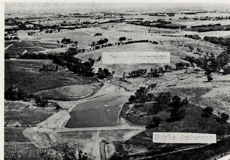
Floodwater retarding structure B-5, Moulton Watershed, located on the Doyle Anderson and Bobby Spurgeon farms, 3 mi. west of Moulton. Farmer applied practices in the watershed area around the structure include graded terraces, contouring, diversions, erosion control structure, pasture renovation and grassed waterways.
