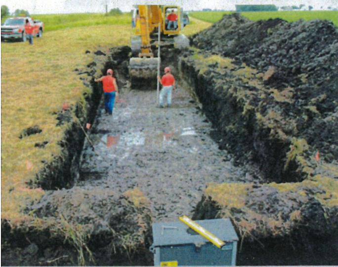
Excavation for a bioreactor: (Courtesy of, Iowa Soybean Association Environmental Programs & Services.)
