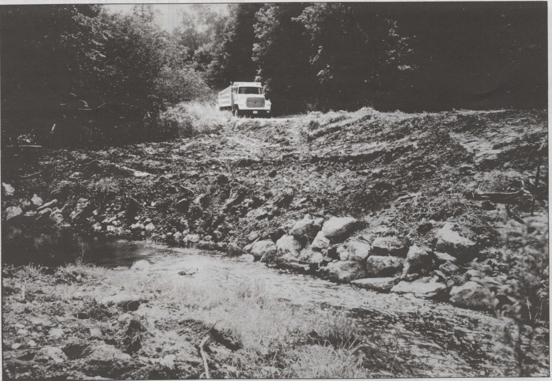
Rock rip rap placed along ditch banks helps to prevent stream bank erosion. Bank hides placed under the rock enhances the stream for fish habitat along with stabilizing the stream bank.
