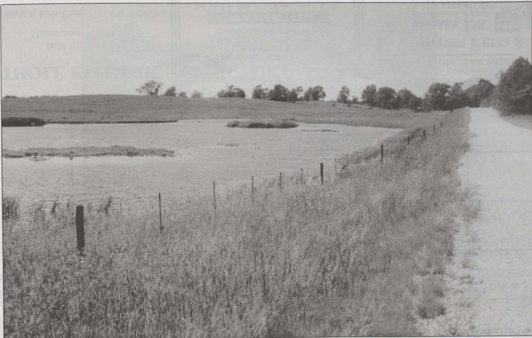
The county gravel road was improved and utilized as the dam for this grade stabilization structure in Spring Branch Creek Watershed. The pond traps the surface water runoff and releases it at a controlled rate to the Spring Branch Creek Trout Stream. The pond also provides habitat for fish and wildlife.
