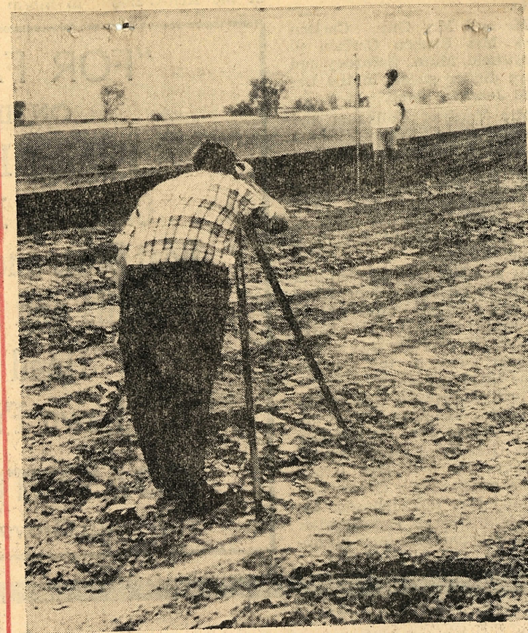
CHECKS — Don Goodenow, SCS, uses an engineers level to check out the completed seeded backslope terrace on the Calvin Goodenow farm. Gregg, Don's son, lends a hand as rodman. The terraces must be large enough to hold a two-inch runoff.
