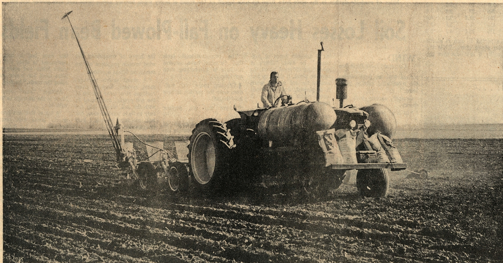
Robert Henning, hired man, plants corn on Feldkamp farm. Each of the two fertilizer tanks on the tractor holds 200 gallons. Bags of seed are stacked on front of tractor.
