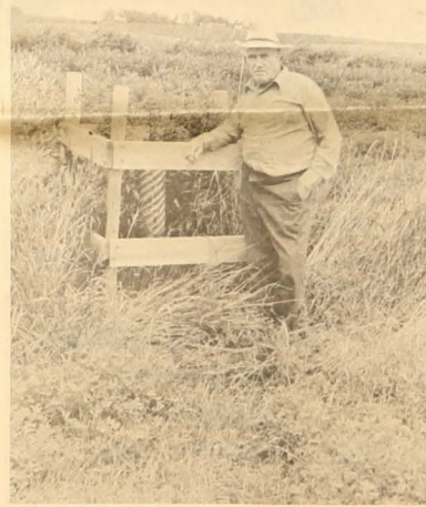
TERACE INTAKE —Odis Rothberger, long-time conservation farmer near Elgin is shown by a terrace intake. Rothberger raises beef cattle. Protection of the intake riser pipe is necessary when cattle are in the field.
