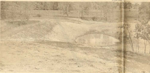
EROSION CONTROL — This erosion control dam with a permanent water pool will provide livestock water on the George McDonald farm in Clermont township. The dam also stabilizes a ditch and will have downstream flooding benefits.
