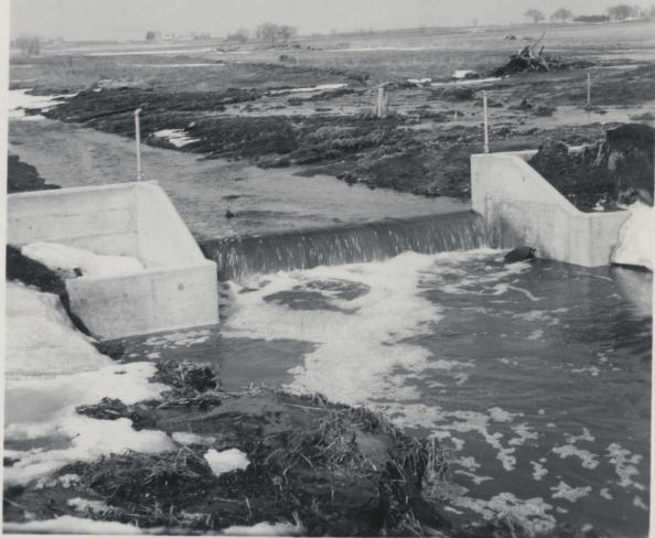
Hoffman/Broghammer concrete structure built Sept. 1959 picture taken 3/31/60
