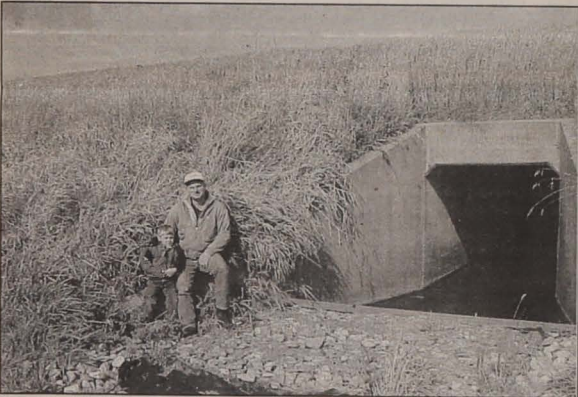
JODY AND JOSEPH KASAL ON THE outlet end of the box culvert. Tile on both sides takes the seepage from the waterway. At high flows, the water will spill out on rock filled baskets.
