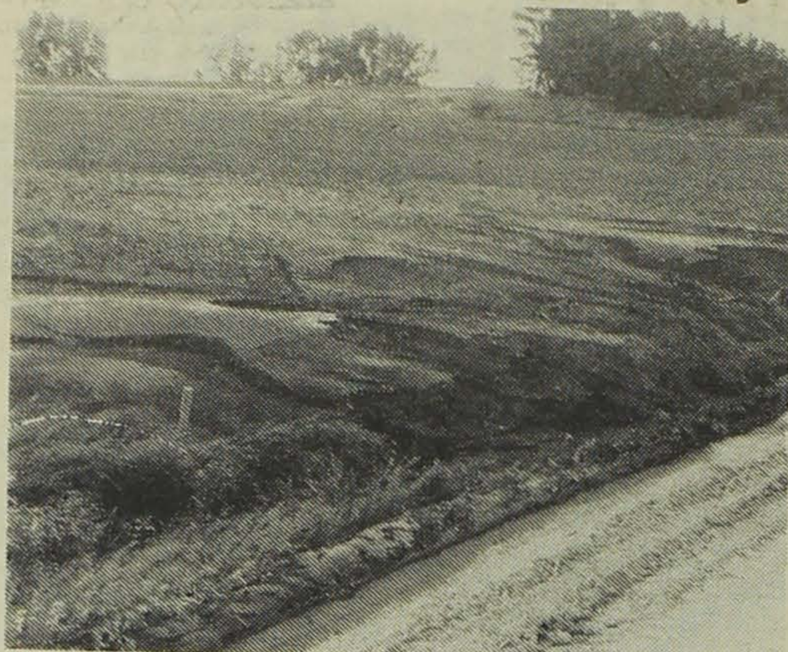
Soil loss drastically exceeded acceptable limits on this Cass County field in 1985. Many simple and low cost conservation practices can be used to reduce or eliminate excessive soil erosion.
