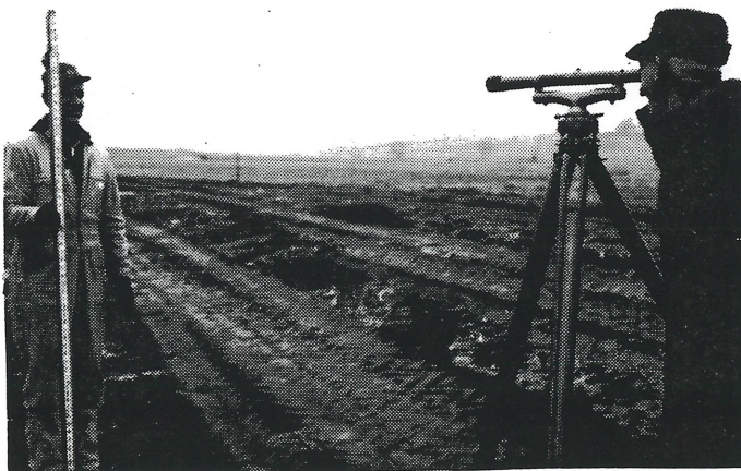
Wayne Rake, Contractor & Dutch Kraft, SCS Tech. check out broad base terraces completed on the Virgil Linman, Robert Mitchell farm south of Arthur
