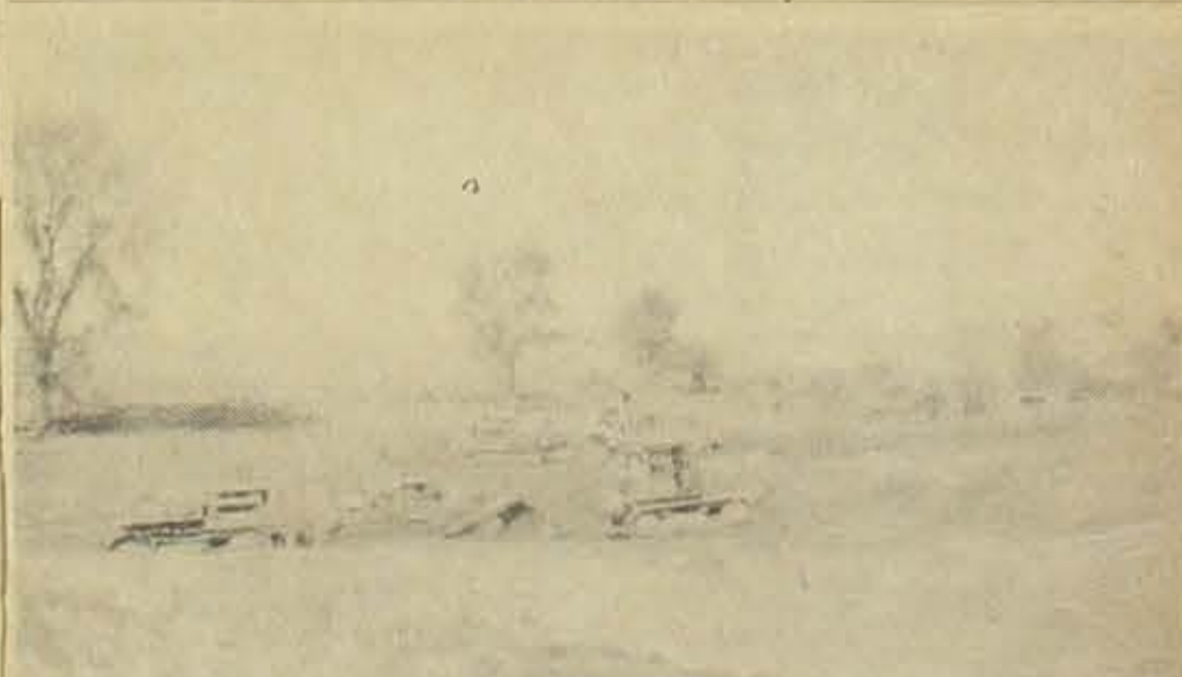
The above picture shows construction work underway on one of several major projects completed as a part of the field day program. Five dozers and two scoops were at work on the above pond, one of three constructed Thursday.
