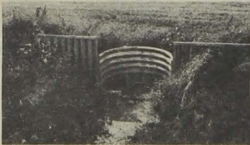
Grade Stabilization Structures - control gullies. This aluminum drop spillway installed by Frank Cook, New Providence, Iowa is one example of a grade stabilization structure.
