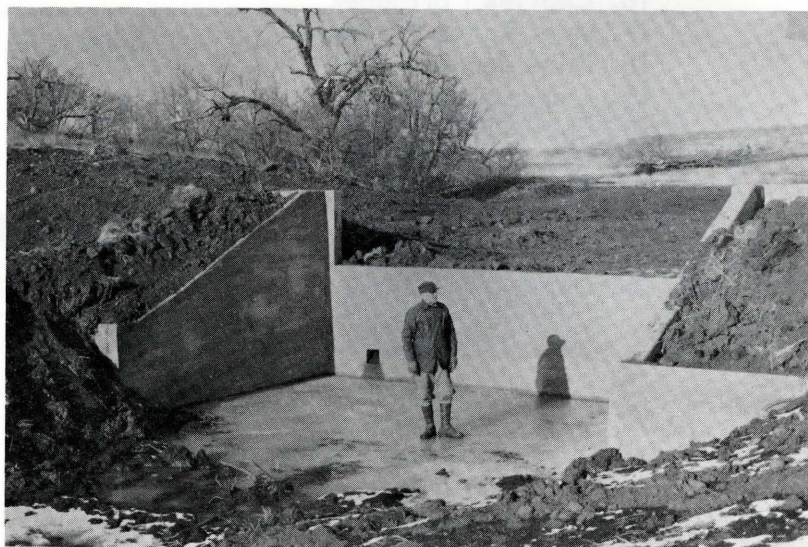
After: Structure, reenforced concrete, 7-foot drop. Ed Allely farm. 33 cubic yards of concrete were used for this structure.
