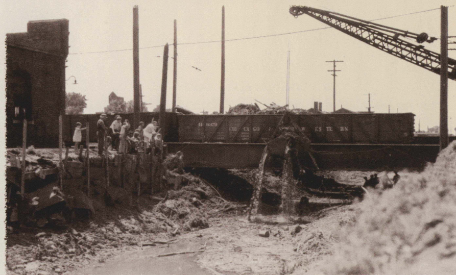
Onlookers observe early-stage construction of the Indian Creek channel improvements near the Chicago & North Western Railroad bridge at 1 st Avenue (courtesy of the Pottawattamie County Historical Society [no date]).
