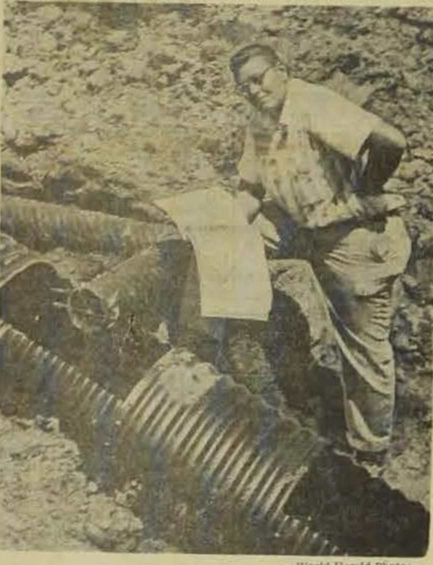
Becker . . . Toe drains insure stability.
