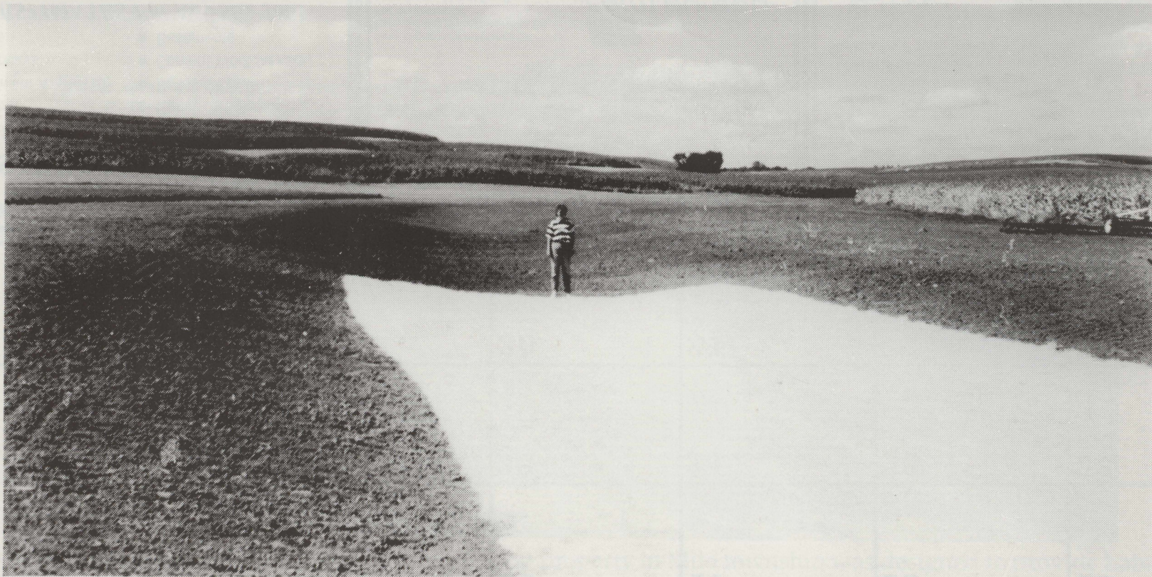
Soil Conservation Technician, Robin Gudenkauf is checking a newly constructed grassed waterway on the Mr. and Mrs. Russell Bradke farm in Union township. A curlex fabric material is used to stabilize the outlet portion of the waterway until the grass cover can become established.
