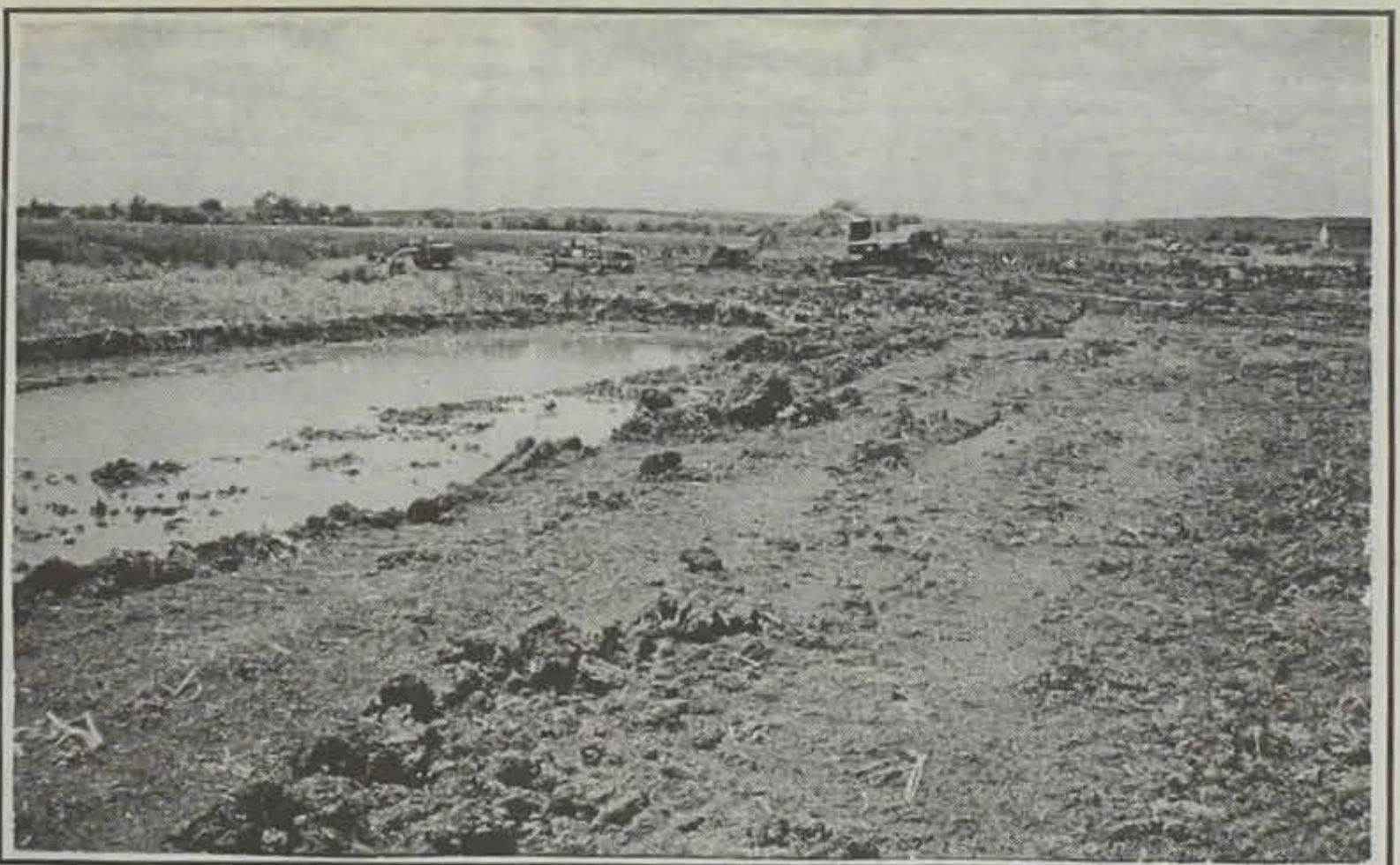
In top photo Ed Christensen, Steve Van Riper and Chris Christensen point out various aspects of their new wetland area as it is being created. In lower photo, Chad Taylor and his crew are busy creating the new wildlife area. The construction work was done in June of this year.
