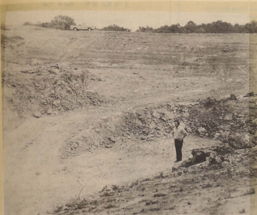
Jim Settles stands in a small silt deposit area, part of the larger silt pond. The dam is in the background, just recently completed as part of the necessary measures in making the Franklin Township Lakesite a reality.
