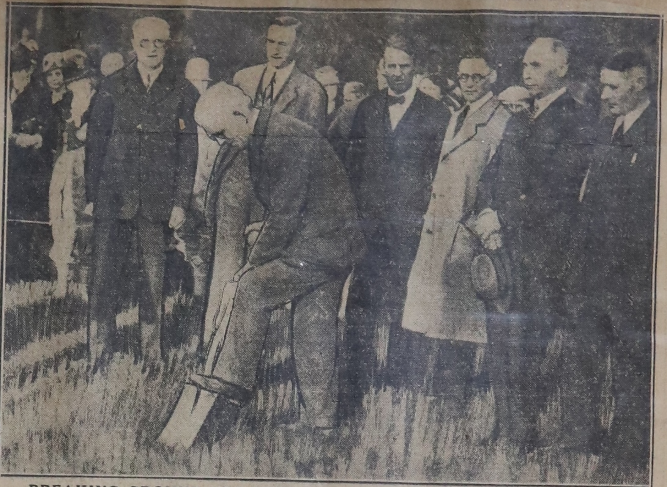
BREAKING GROUND FOR NEW CHURCH. Dr. Burtis R. MacHatton cutting the first sod for the new Plymouth Congregational church on Ingersoll avenue between Forty-first and Forty-second streets. With him, left to right, Harry B. Lewis, Charles E. Lynde, Dr. F. N. Ralston, W. P. Bair, D. D. Needham, F. M. Cline.
