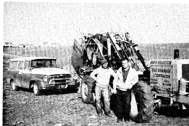
Bill Olson and Dick Ahrens of Conroy are shown just finishing another tile job on the Frank Ahrens farm in Hilton Twp. Bill and Dick work for Olin Helgeson.
