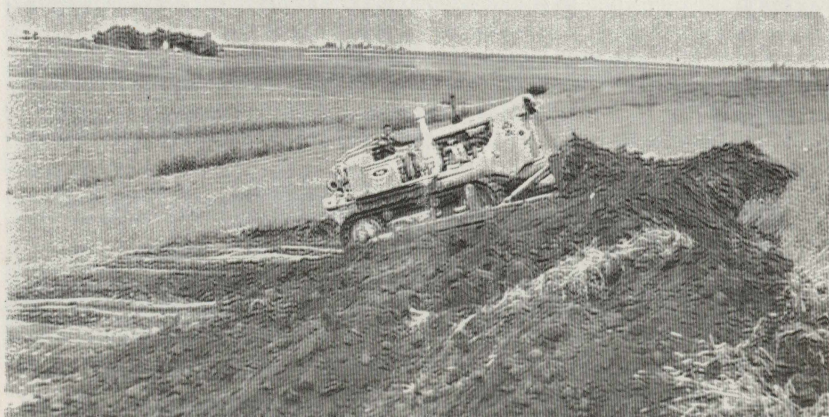
Bulldozer building grassed backslope terrace. Notice how the slope is flattened below the terrace. The 2:1 backslope is seeded to brome grass.
