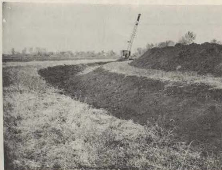
An open ditch being constructed during October, 1967 on the Jerry Wolf farm.
