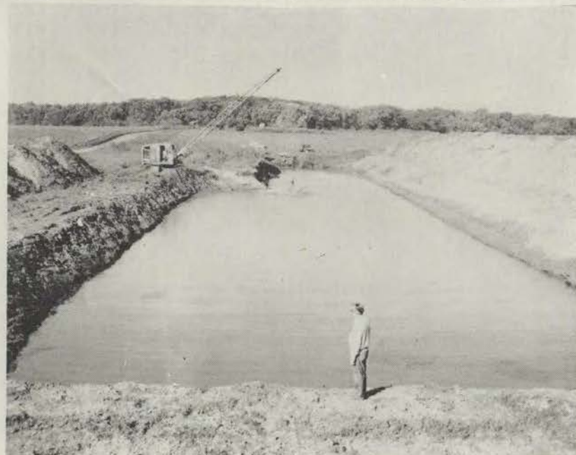
Erpelding's pit pond under construction during October, 1967.
