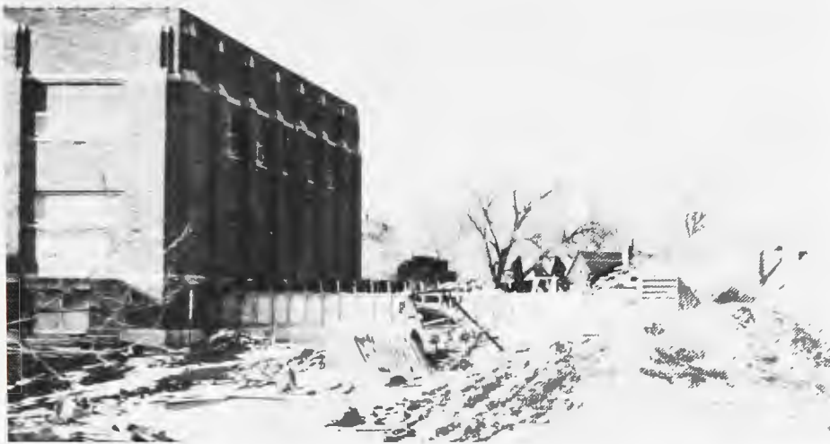
Work was started on the new gym.
