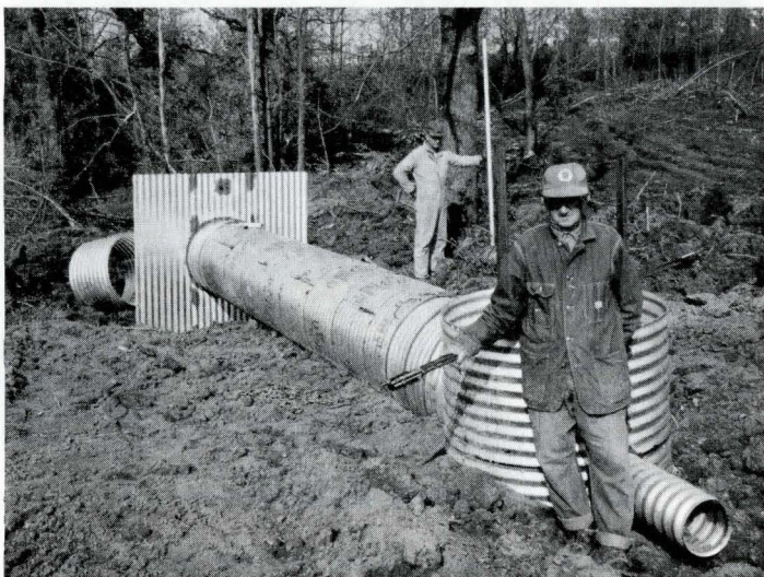
Walter Fritz, foreground, and Charles Bruggmeyer, contractor from Mt. Pleasant, Iowa are shown assembling the pipe assembly for a large pipe drop inlet structure built by Walter on his farm in Union Township.
