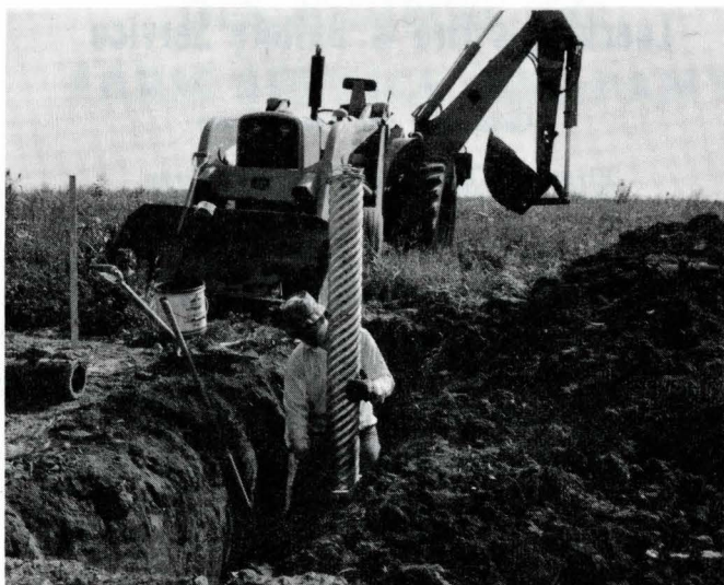
Terry Conrad working for Allgood Construction is shown installing a terrace inlet pipe on the Helen Williams farm, operated by Louis Bloomberg in Union Township. Twenty-one such inlet pipes were installed.
