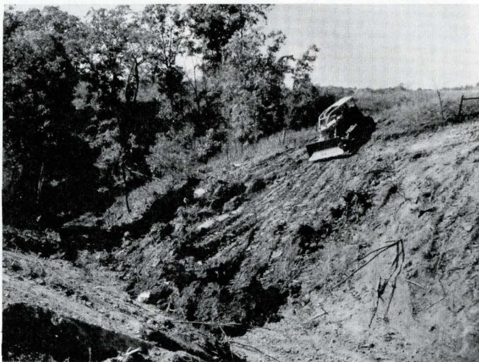
Chuck Allgood, contractor from Winfield, Iowa is shown stripping the dam site for a large pond built by Wm. Gerdes in Tama Township. About a mile of tile inlet terraces were built in this field at the same time.
