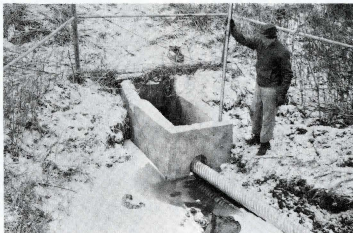
A small drop box on a road culvert is being checked by Sandy Hedges of the SCS. The box built by contractor, Franz Charbonneaux of Burlington, is located on the Jack Inghram farm in the Geode Watershed. The engineering design for this box and the large dam on the Taeger farm above was provided by the Area Engineers located in Fairfield to service this area.
