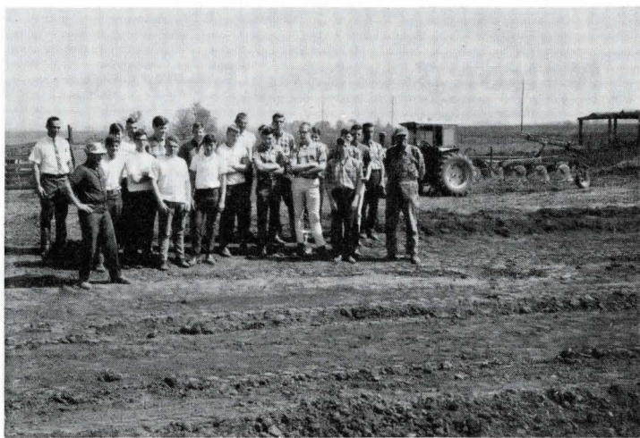
The Mediapolis FFA class and their instructor, Jim Howell, visited the S. S. Barton farm in Yellow Springs Township, to watch the disappearance of ditches and the construction of over a mile of tile inlet terraces last May. Barton, standing to the right is ready to start plowing the straight terraces with his big 5 bottom outfit.
