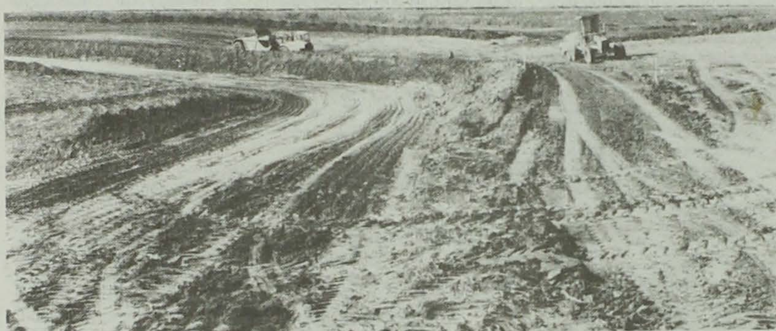
Large earth moving machines are shown as they are used to build grass back terraces on a Cass County farm. (Photo furnished)
