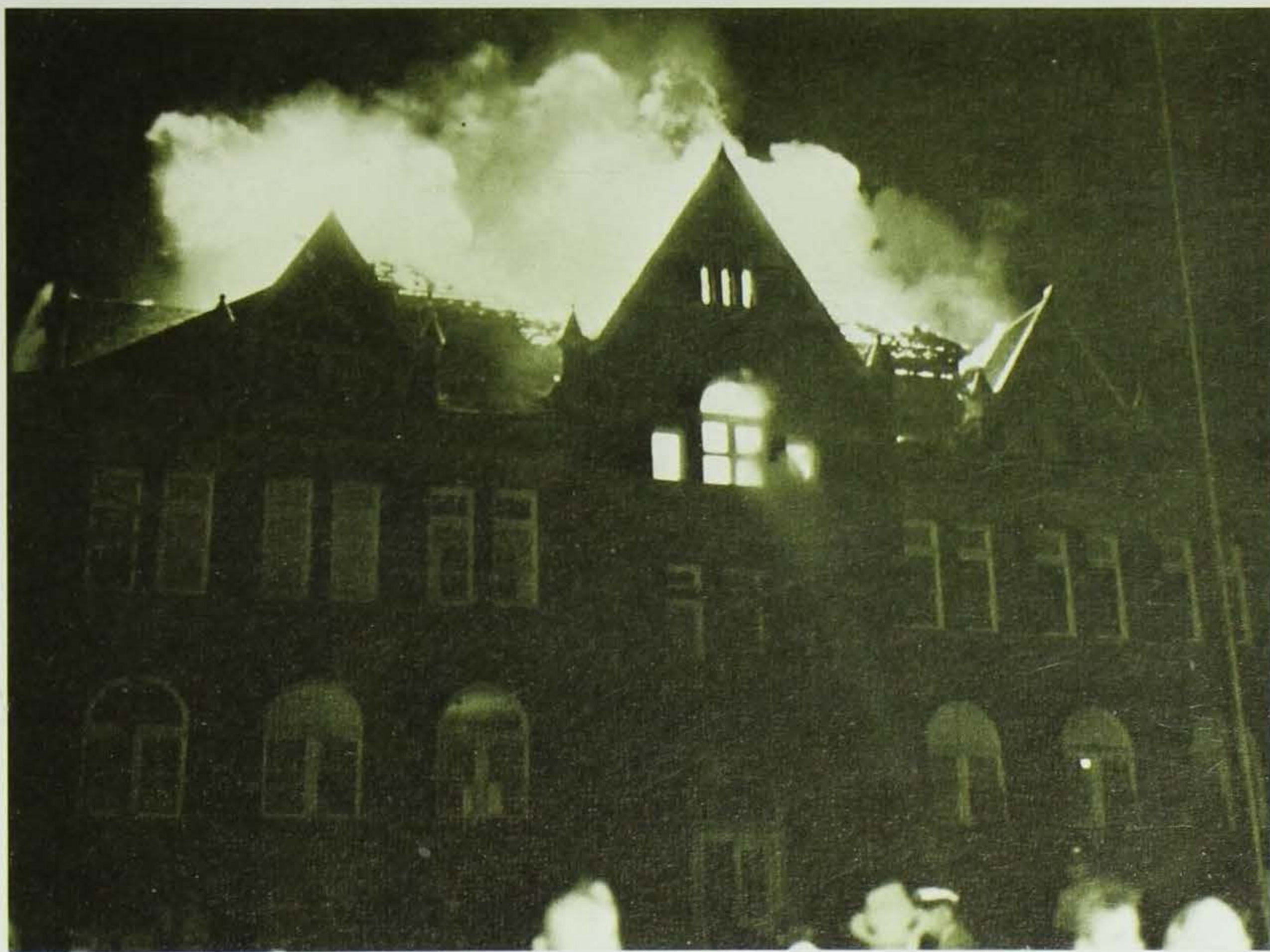
A fire destroyed the building on September 27, 1956; it housed all the administrative offices, theater, and almost all
