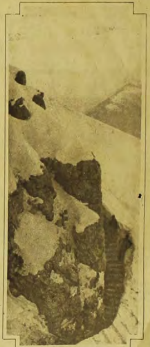
A Section of Italian Communicating Trench Which Runs Along the Mountain Peaks on the Asiago Front
