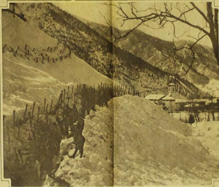
Italian Soldiers Building Barbed Wire Defences and Intrenchments Along the Steep Mountain Sides
