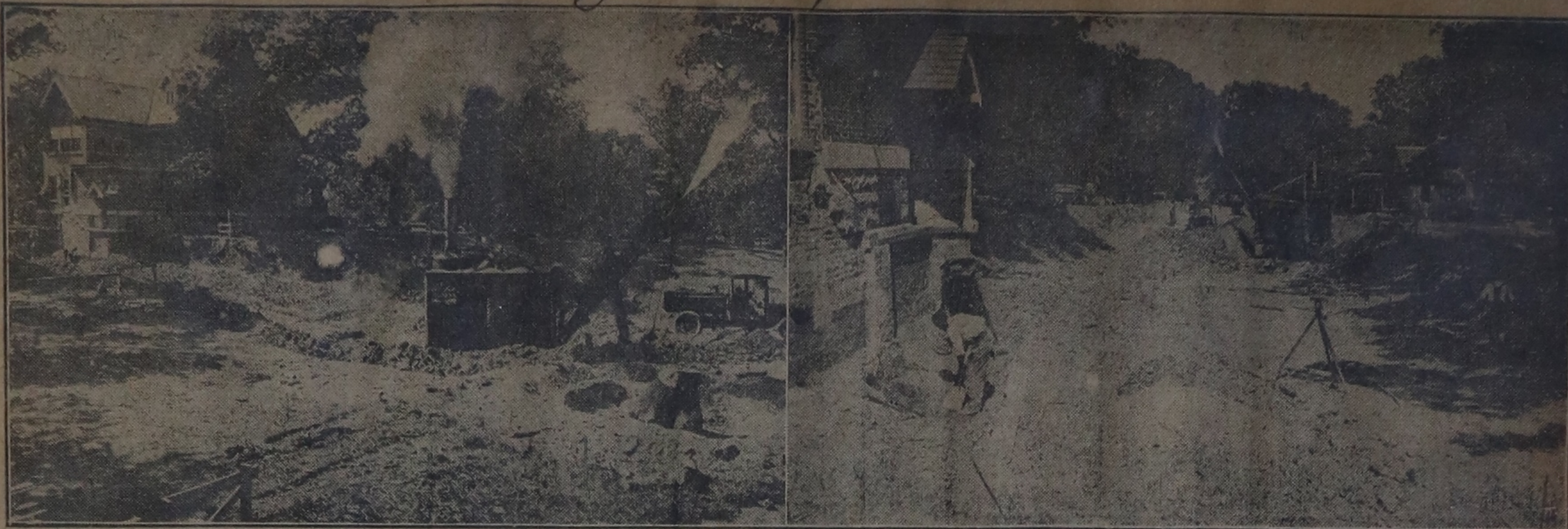
NEW CHURCH CONSTRUCTION. Two views of the excavation work for the new Plymouth Congregational church which is to be erected on Ingersoll avenue between Forty-first and Forty-second streets. —Schwartz, Evening Tribune Photo.
