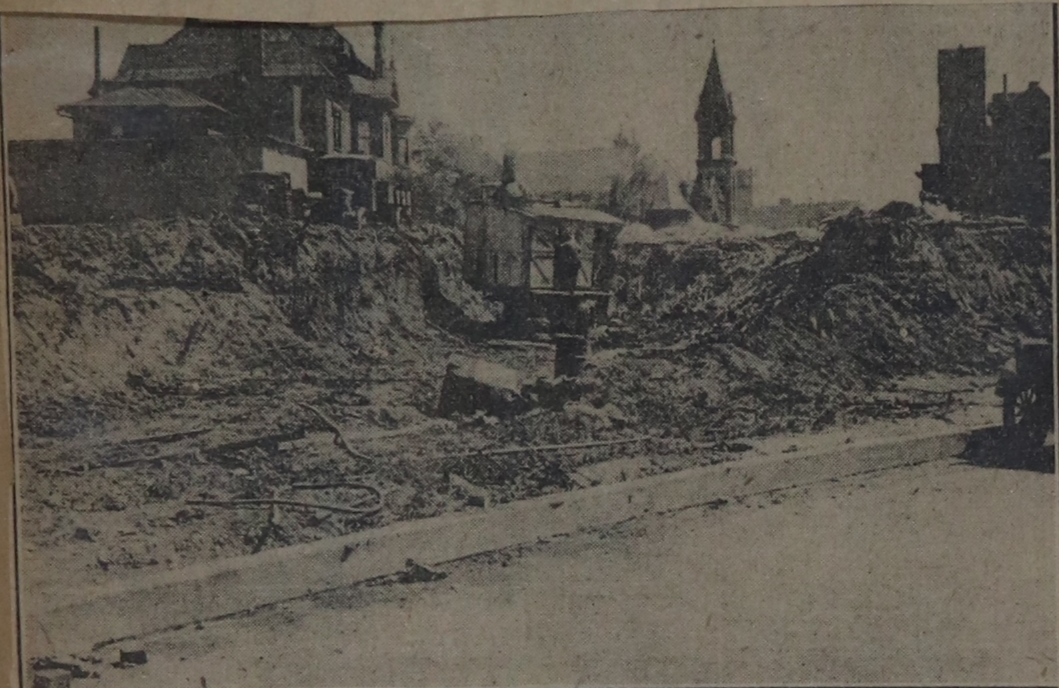
DIGGING THROUGH EIGHTH STREET. The beginning of grading down Eighth street from the Keosauqua way end.
