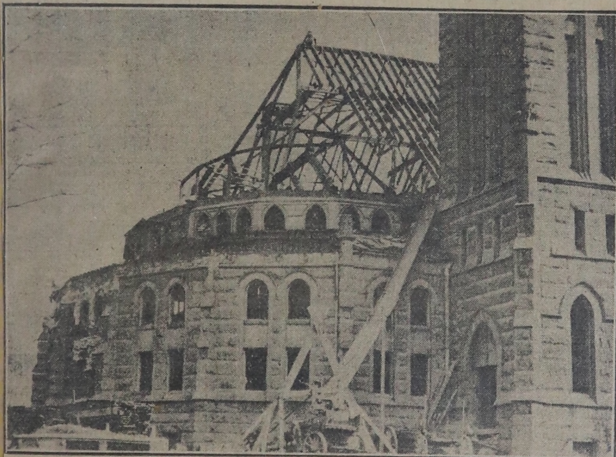
—Evening Tribune-News Photo. FAST WORK. The work of wrecking the Plymouth Congregational church is proceeding rapidly. This picture shows progress made on the job.
