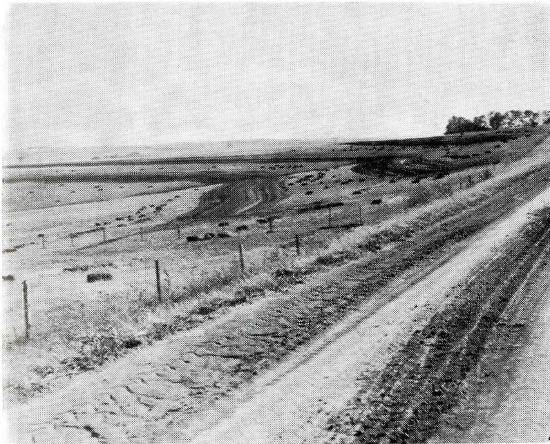
Standard terraces constructed on the Randall Baier farm in Noble Township. Fall 1959.
