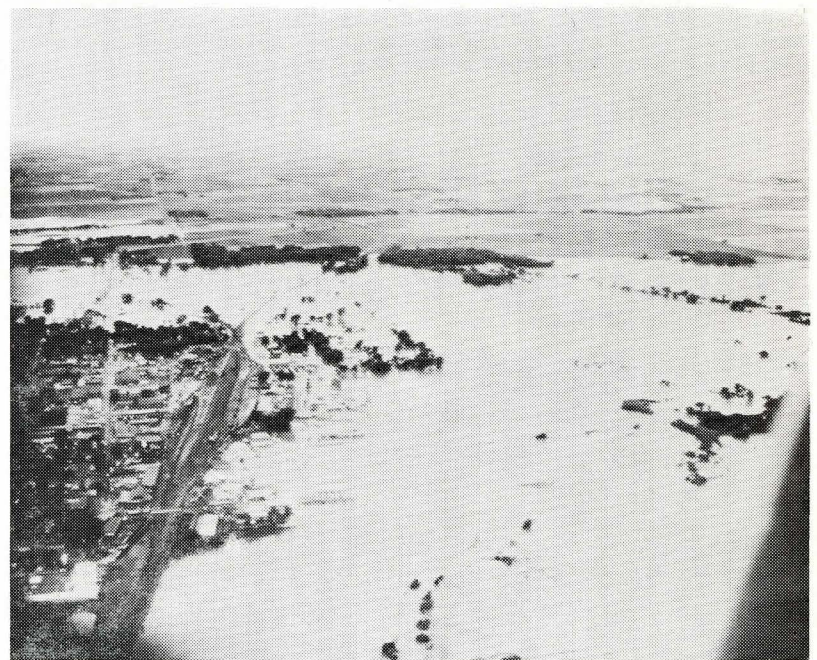
View looking west at the north edge of Atlantic during the height of the July 2, 1958 flood.
