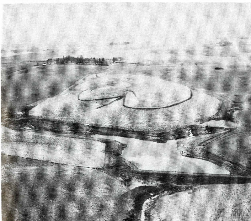
One of the outstanding recreational spots in Cass County where a two-acre pond was established by the installation of an earth fill with a drop inlet. The Conservation Commission has assisted with the development of this area for wildlife protection and recreation.
