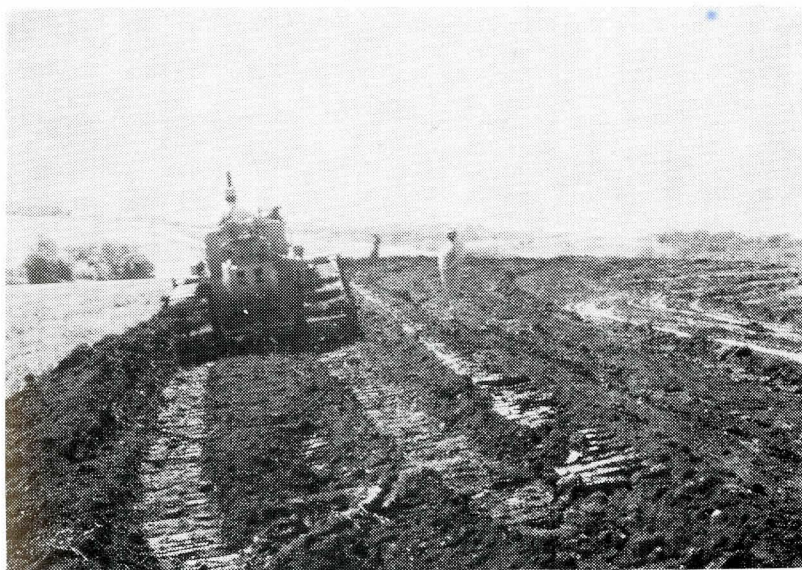
This is the first parallel terrace constructed in Cass County, on the Tom Burns farm. Field Day, fall of 1958. Picture shows caterpillar constructing long farmable slope on the terrace. This terrace is designed for the use of four-row equipment.
