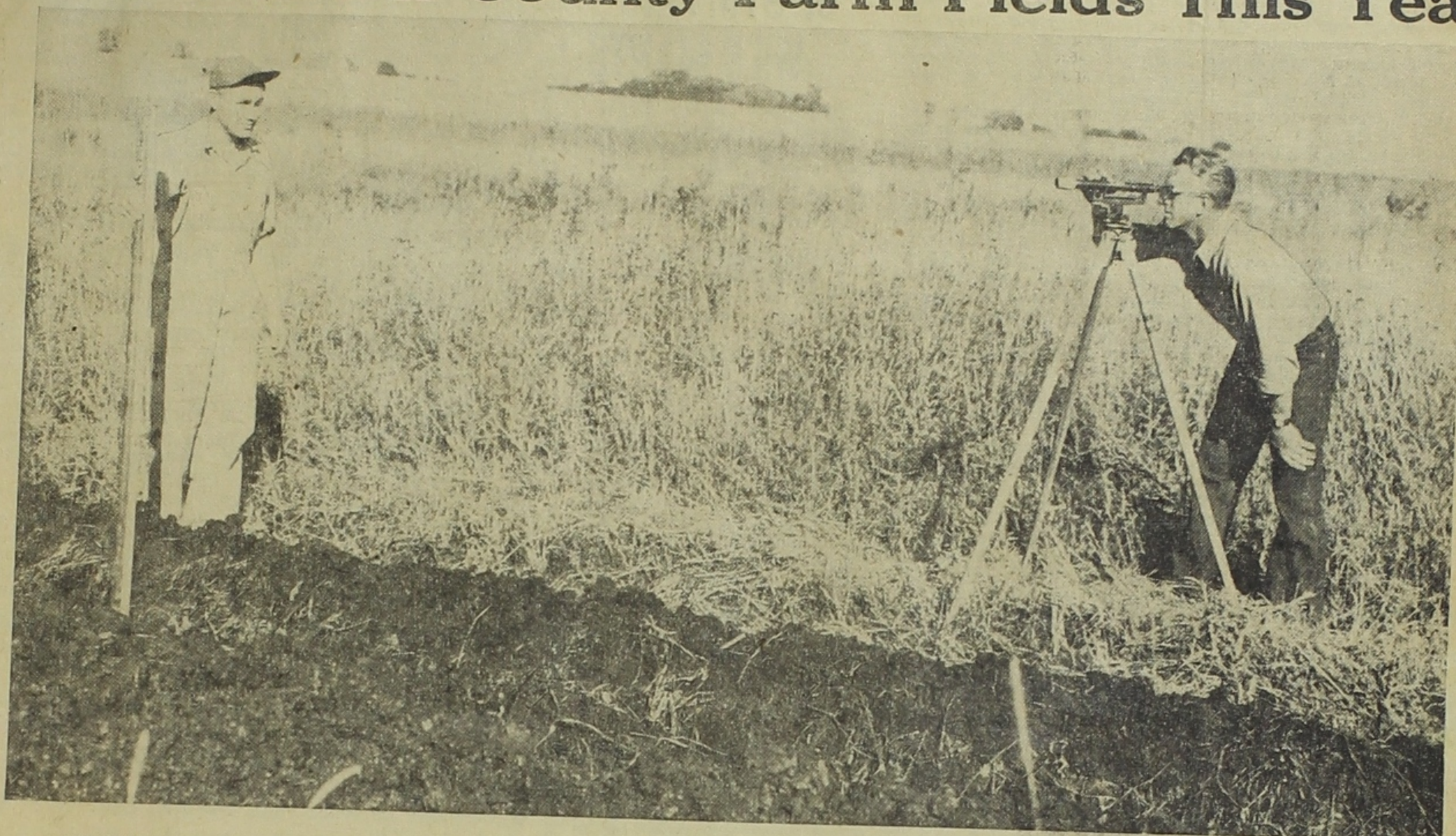
CHECKING THE GRADE of tile being laid at a farm operated by Archie Dunkelberger 2 1/4 miles northwest of Mt. Auburn are Clarence Byer, left, and
