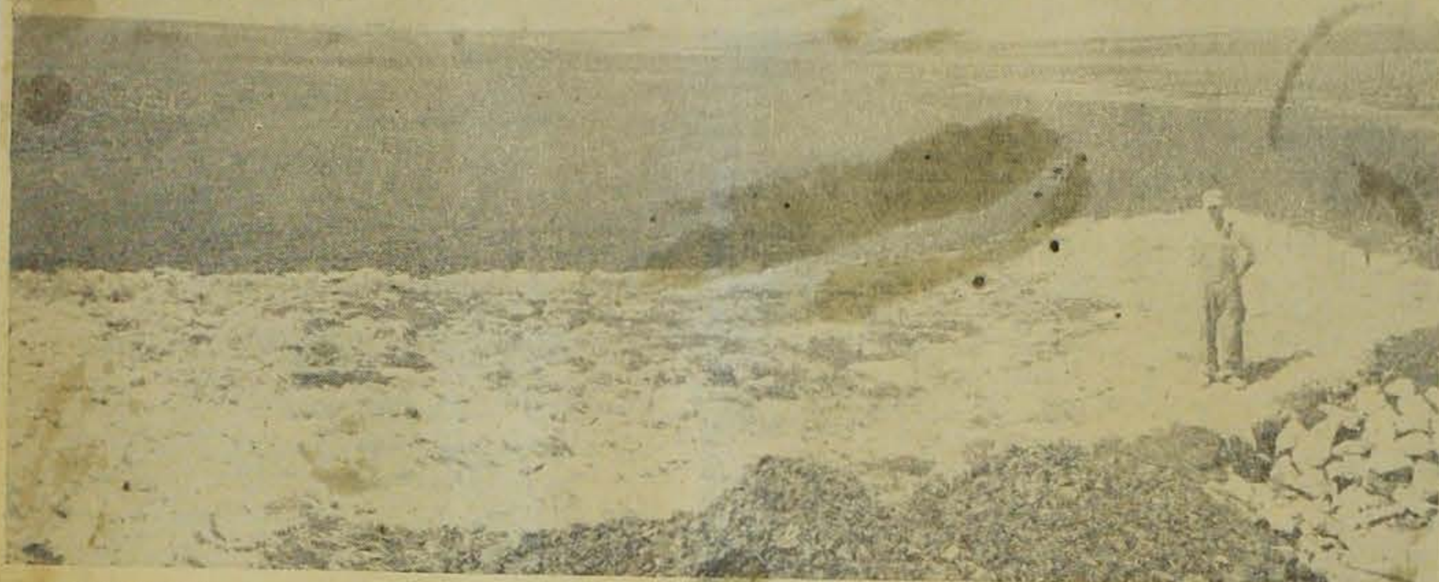
JACK FRY, hired man on the 260-acres owned by Oscar Olson and farmed in partnership with his son, Arthur, four miles south of Vinton, stands at the edge of an inexpensive rock and sod flume at the mouth of a new waterway on the place. The waterway got rid of a deep gully that not only washed away rich soil, but also cut a big field into two sections, thus hampering farm operations. Below the big waterway, dish-shaped, is shown with the flume on the extreme left. See story.
