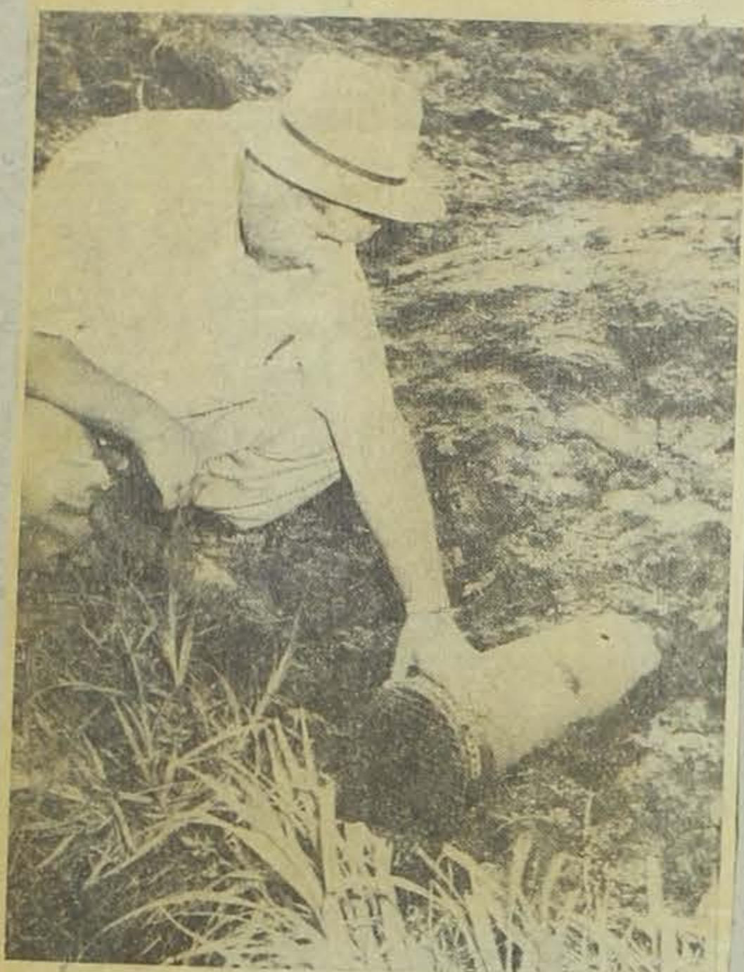
DARREL C. RACE inspecting Benton county tiling project.
