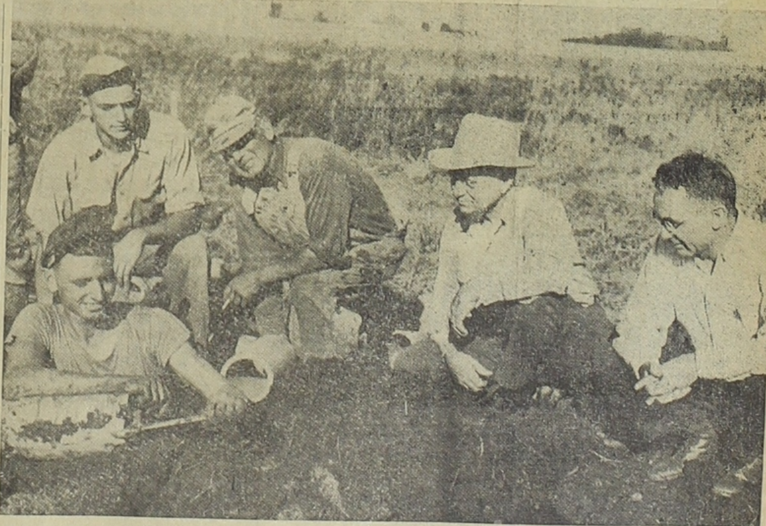
TILER OTIS HILMER works on a junction of two lines of tile on the L. J. Robertson farm near Mt. Auburn as farm operator Archie Dunkelberger, helper Tom Winters, PMA committee-man Earl Wallace and conservationist Glenn Heady watch.
