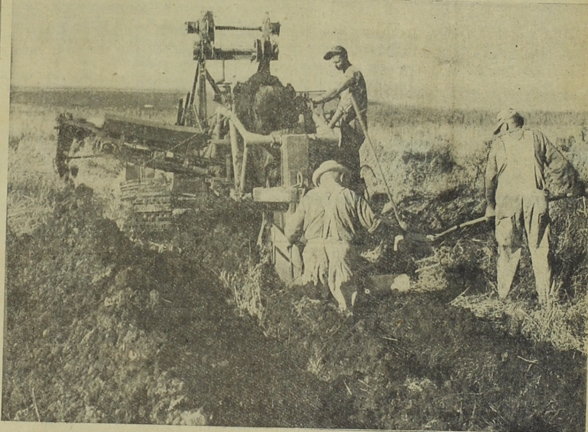
DIGGING TRENCHES and laying tile is done in the same operation by Otis Hilmer of Dysart and his two helpers, Tom Winters and Claus Mueller both of Dysart. While Hilmer operates the digging machine, Winters keeps Mueller, who places
