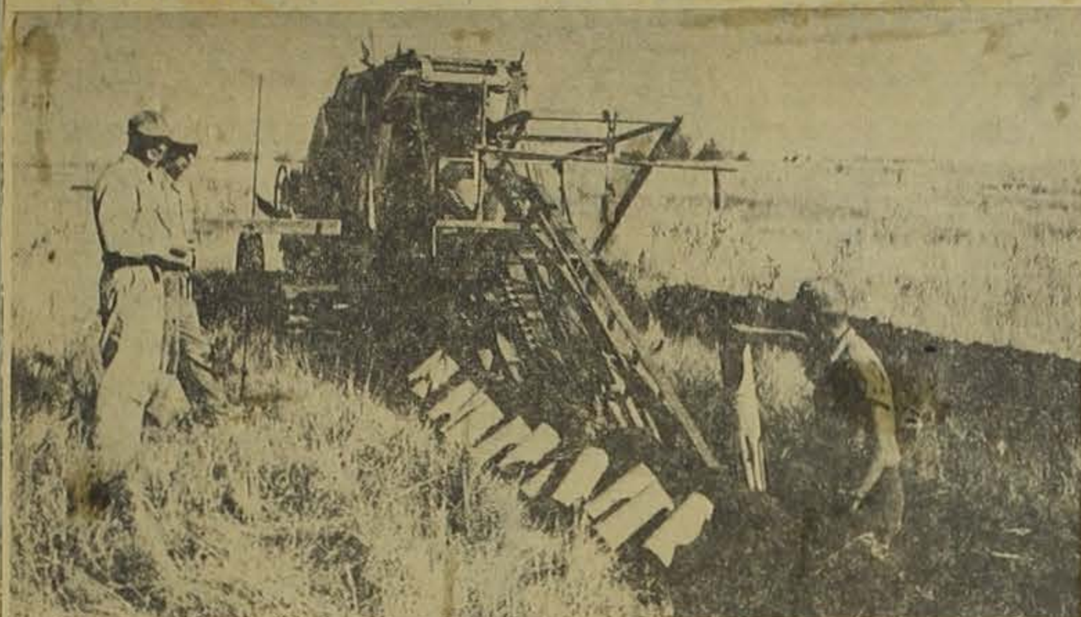
A TILING MACHINE lays 4,000 feet of four and six-inch clay pipe in a 35-acre field belonging to Henry Boddicker. The piece has never been cropped. —Daily Times Photo-Engraving
