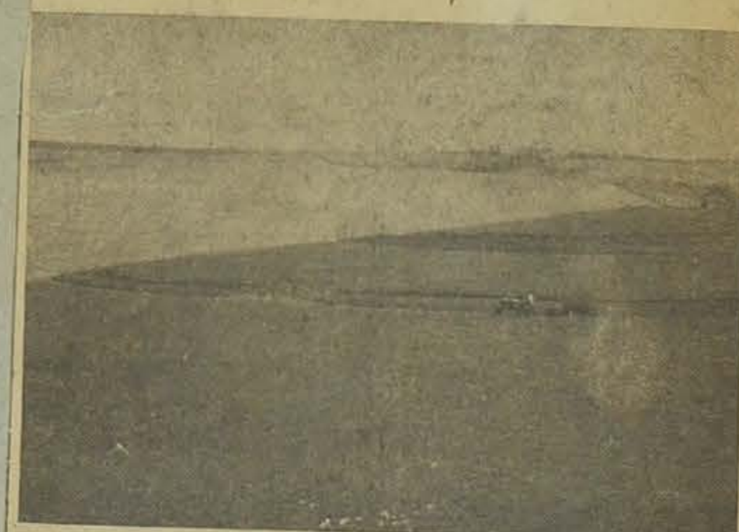
THIS AERIAL PHOTO shows how terraces have been constructed on the Orrin James farm. A whirlwind terracer was used for the conservation project.
