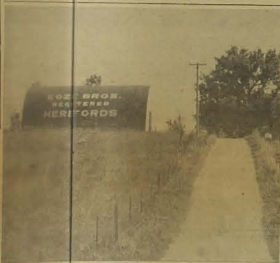
THIS RED QUONSET HUT WITH THE WHITE LETTERING is familiar to all travelers who pass the Kozik farm on U.S. 30 north of Belle Plaine.
