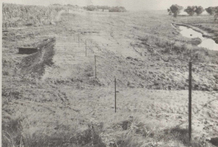
Gully Control Structure on Harold Bahl farm in Silver Lake twp. consisted of 50' of 21" diameter pipe for barrel and 6' of 30" pipe for the riser. The riser is also used for a tile outlet. Also 950 cu. yds. were used for the earth fill and shaping the waterway above the earth fill.
