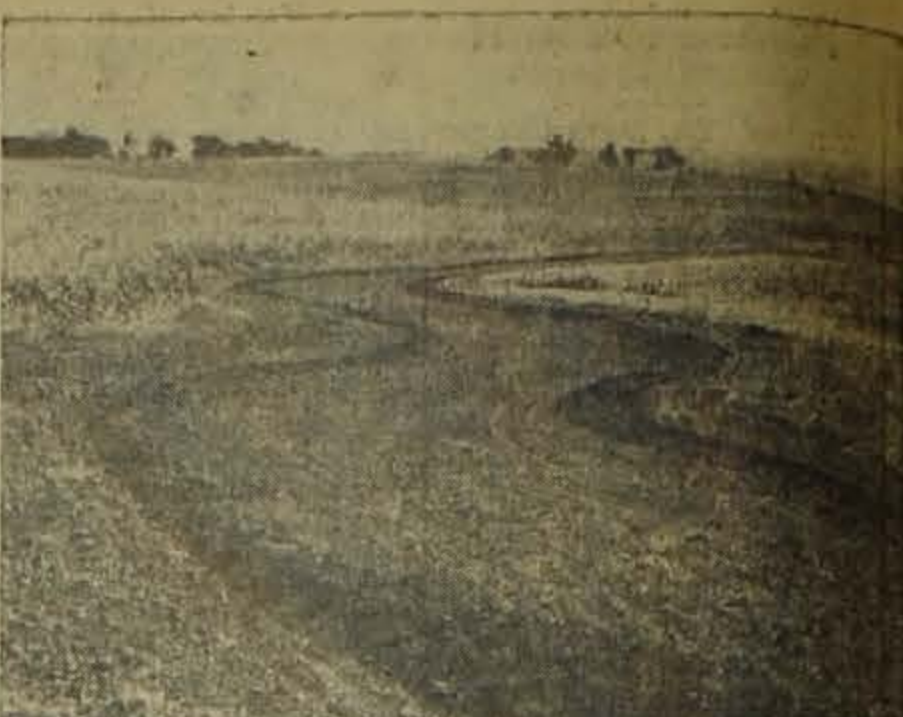
A newly constructed roadway to be seeded to permanent grasses. Grass waterways allow safe runoff during hard rains without excessive washing.
