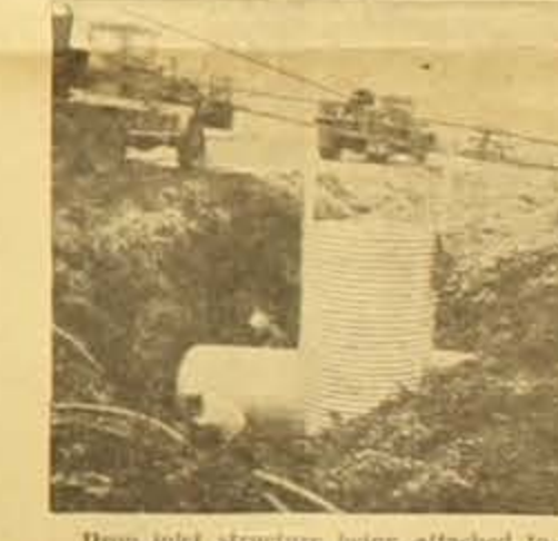
Drop inlet structure being attached to road culvert through joint efforts of farmer Rex Brown, County Board of Supervisors, ASCS and SCS.
