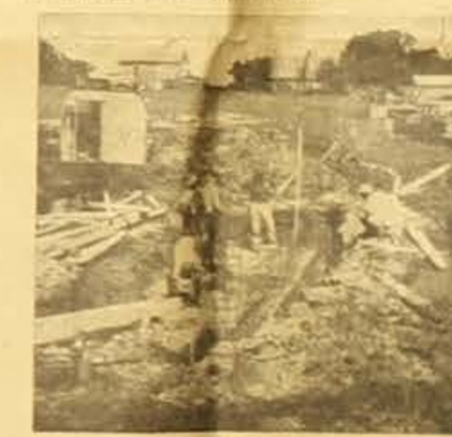
Concrete, steel and inspection of a gully stabilizing structure near Jamaica.
