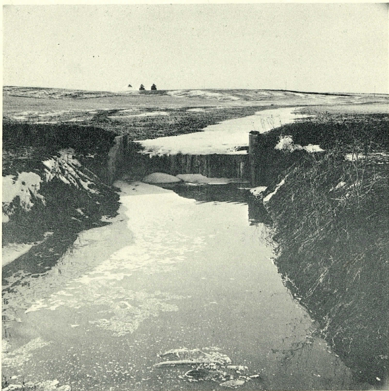
Water running through the dam and waterway built on the Mrs. Pogue Sherrill farm, 2 miles south of Tipton. Tile were also installed alongside the waterway.
