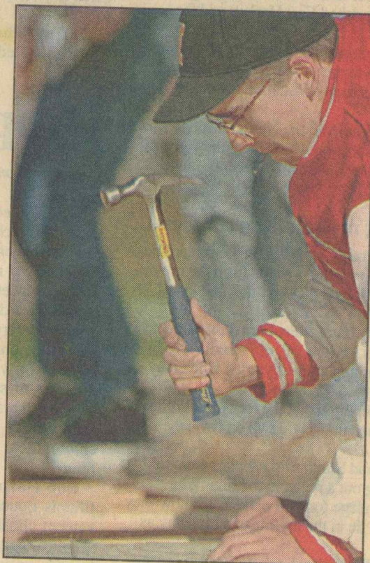
Hammer in hand and nail in mouth, Zach McLean helps lay down flooring.
