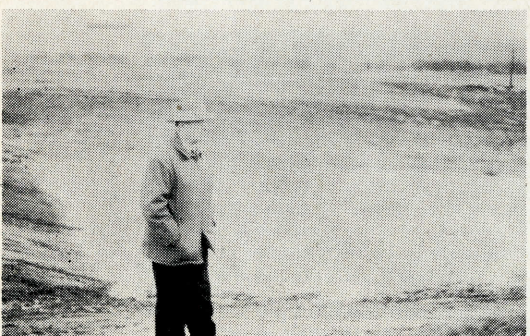
E. E. Smith, SCS Area Conservationist, Chariton, Iowa, inspects the John Mitchell structure 2 miles north of Centerville. Permanent pool will be 1.56 acres and above that will lie 9:00 Ac. Ft. of temporary storage.
