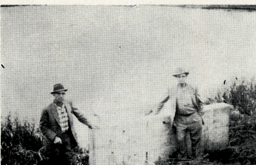
Appanoose County Board of Supervisors, Lee Benz, and Glen Johnson, inspecting the Gilford Davis drop inlet structure southeast of Russell, Iowa. This 7 acre permanent pool is one of 21 similar structures in the Honey Creek Watershed.
