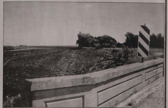
A parabolic waterway was constructed in Washington Township using EQIP funds.
