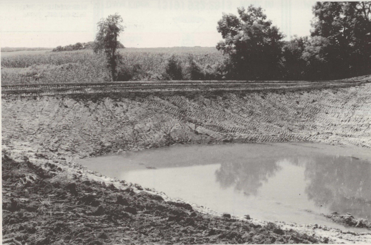
Water and sediment control structures reduce run-off and provide protection down stream from flooding and soil erosion. This newly constructed project in Delhi Township will also provide water for fish and wildlife when the pond area has filled.
