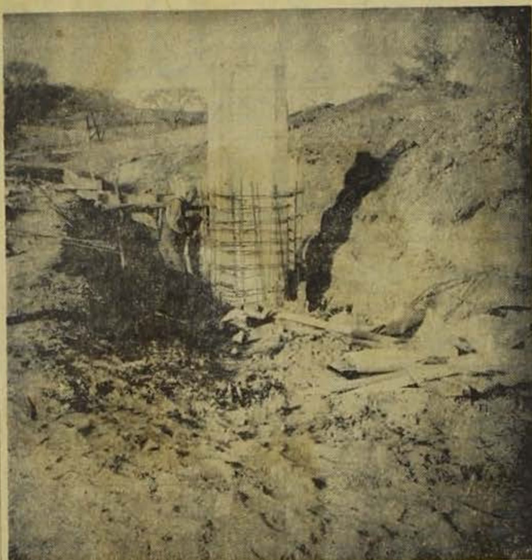
Lud Johnson is pictured at work on construction of the riser of the drop-inlet overflow for the new Monroe County Farm pond. Surplus water drops through the riser into the pipe pictured below.
