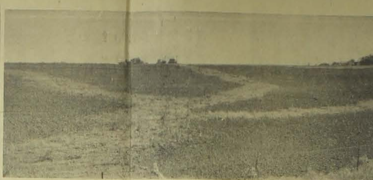
The light-colored areas in this photo show natural grassed waterways on the 240-acre Harold Gardner farm in Bluff Creek township. The waterways serve as terrace outlets—about half of Gardner's cropland is terraced.
