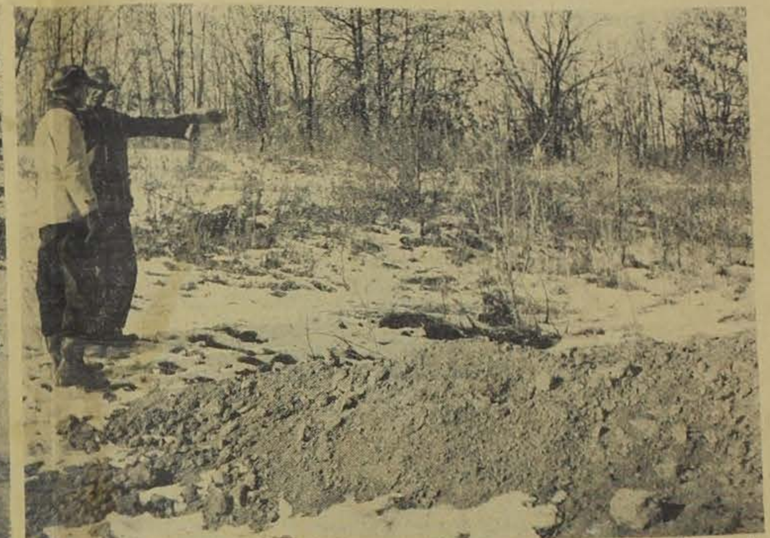
Smith points out to Botts the silting basin he is building above his pond site. The small dam for this basin is the bank of fresh dirt in the foreground. A tile outlet from this dam will take clear water into the big pond.
