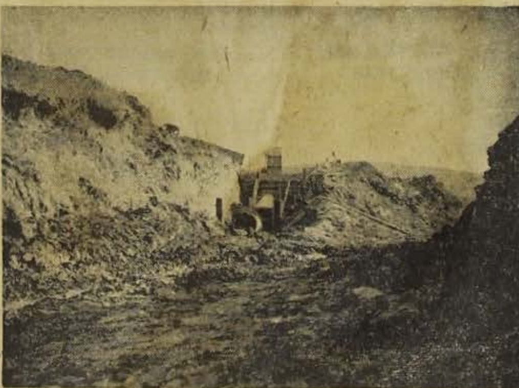
Here's the emptying end of the drop-inlet overflow, shot from the bottom of the gully the project will eventually heal. A dam of 3000 cubic yards of dirt will cross the ditch, and the overflow pipe will run beneath it.
