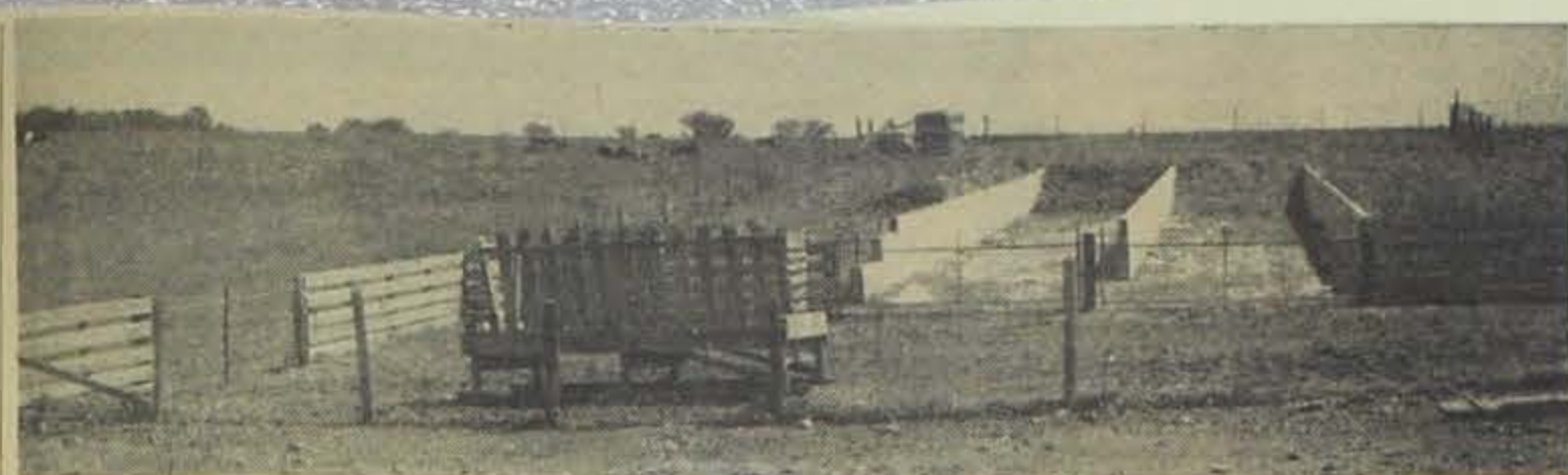
Good land produces good livestock feed, and it must be conserved following harvest to bring maximum efficiency in dairy and beef feeding operations. Pictured here are permanent pit silos, built of concrete, on the John Goode farm in Jackson township, operated by Don Richards. A Holstein dairy herd will utilize the feed stored in the silos. There's an improved alfalfa-brome pasture in the background at left.
