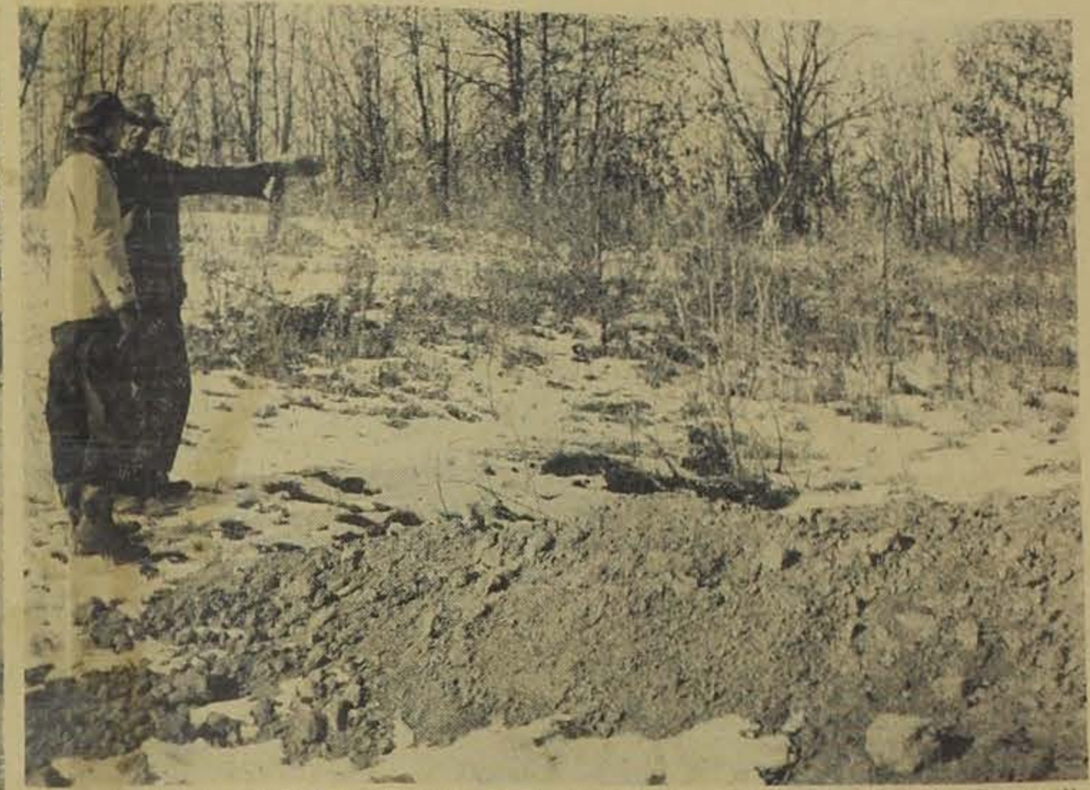
Smith points out to Botts the silting basin he is building above his pond site. The small dam for this basin is the bank of fresh dirt in the foreground. A tile outlet from this dam will take clear water into the big pond.
