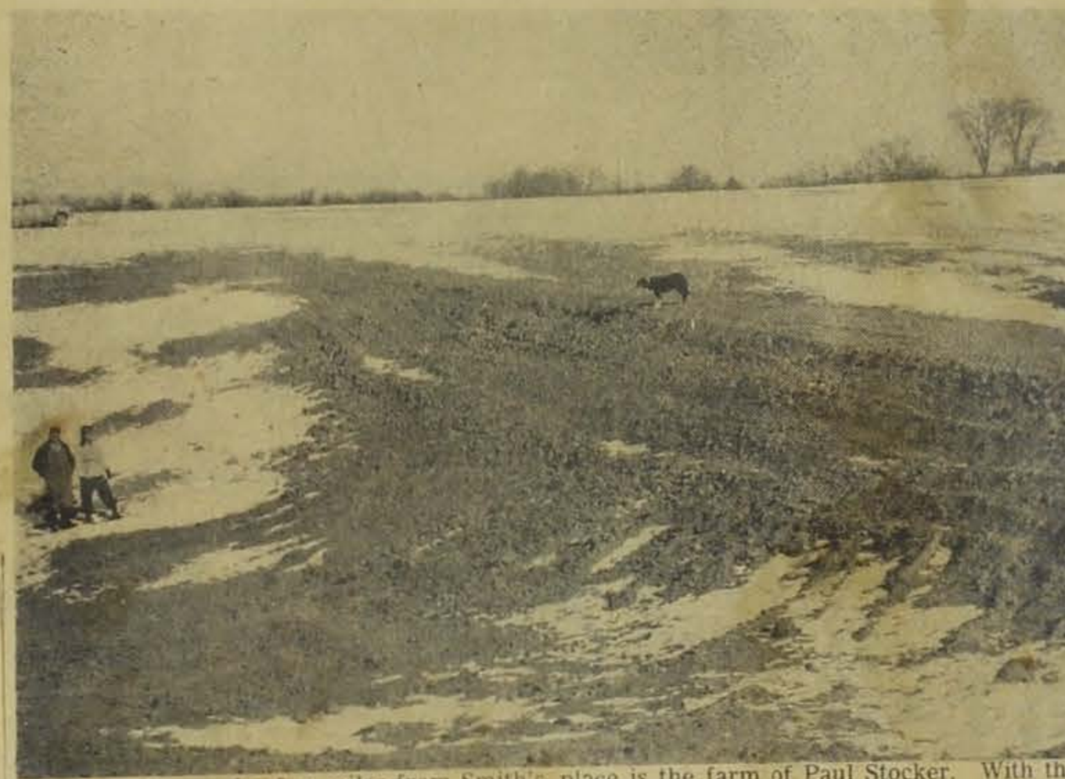
Down the road a few miles from Smith's place is the farm of Paul Stocker. With the help of a neighbor, Stocker built a dam to hold his pond on a site where the soil is clay and water loss through a shale fault is not likely. He doesn't expect to find it necessary to widen his fill in future years, since 3-to-1 slopes were used on the upstream side and 2-to-1 on the downstream side. Picture shows Stocker (left) and Botts at the base of the dam. The dog is at the top of the dam.
