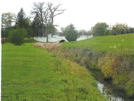
NW tributary south of bridge
