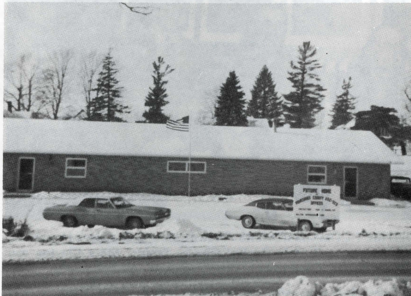
Pictured is the new building in Malcom, which houses the offices of ASCS, SCS and the Poweshiek County Health Services. Sanitarian
