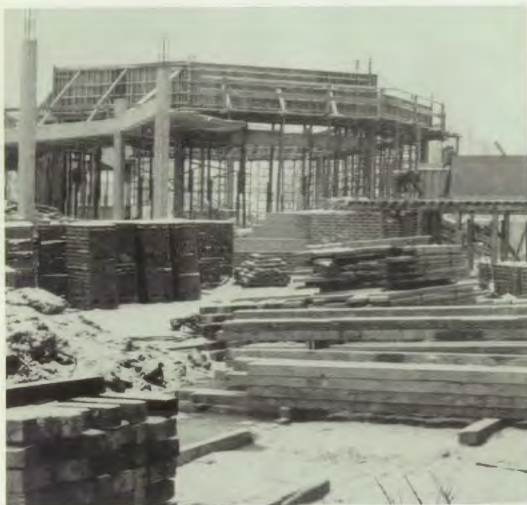
One of the many things happening in Ottumwa for 1978 is the construction of a new Vocational-Technical Building for OHS.
