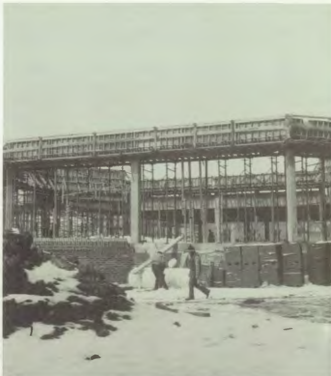
The new Vo-Tech. building was nearly finished in 1978.
