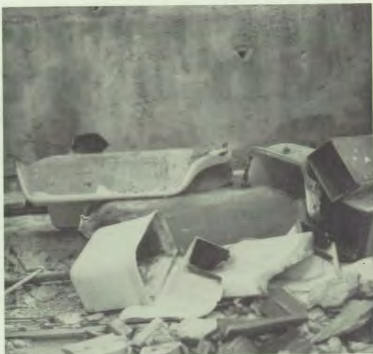
A major project of Student Council is the remodeling of several bathrooms.
